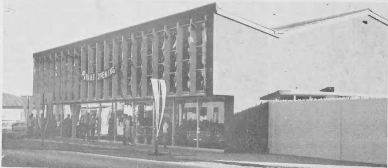
FRONT AND side view of Winkel Handel's new garage and showroom on Bernhardstraat, San Nicolas.
